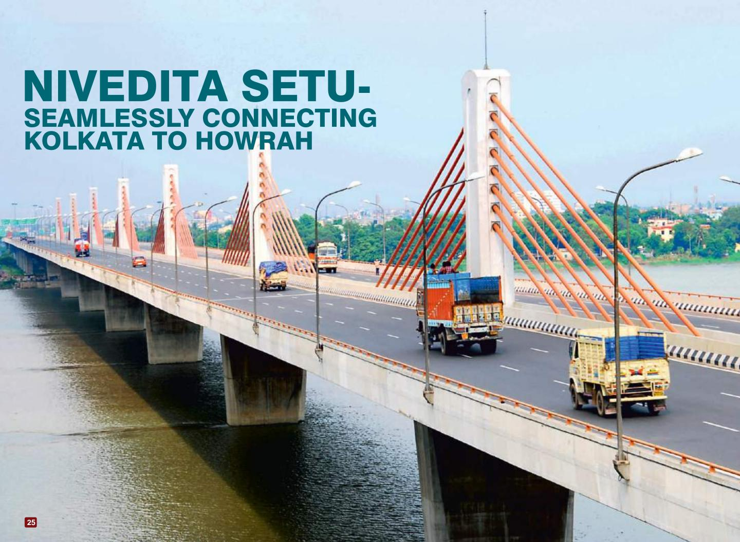
Nivedita Setu over Hooghly River is the first multi-span, single-plane cable supported extra-dosed bridge of India. Completed in 2007, 880 m long six lane with a 2 m shoulder on each side supported by a single plane of stay cables along the median connects Howrah with Kolkata and acts as a gateway to the capital city of Kolkata.
