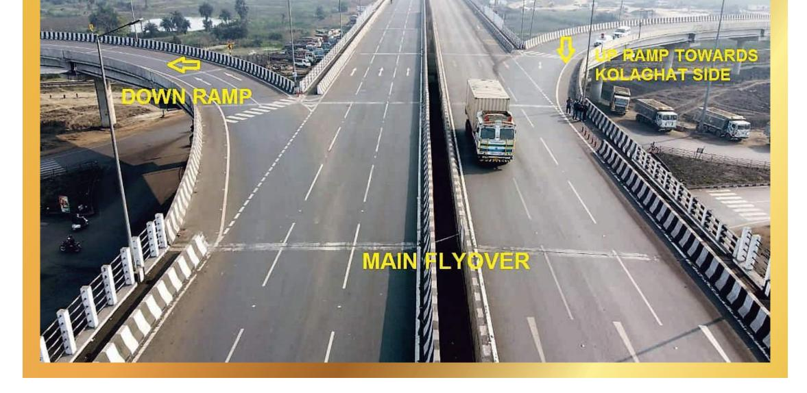
To remove the hassle, construction of 1.4 km long 'Railway Over Bridge Cum Flyover' at Ranichak, built at a cost of around Rs. 190 crores was completed in December 2020 and was opened for traffic from NH 41 to Haldia Dock Complex main gate and vice-versa. The ramps provide uninterrupted flow of traffic for the Port bound traffic from Haldia Township and Durgachak to port.
